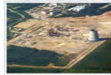
Leningrad Nuclear Power Plant II under construction on 20 July 2010 [3]
